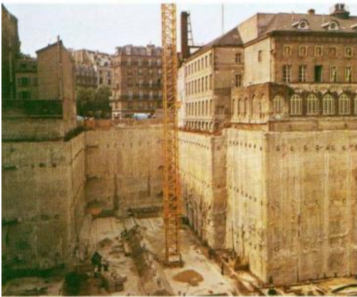
Concreting of the infrastructure
